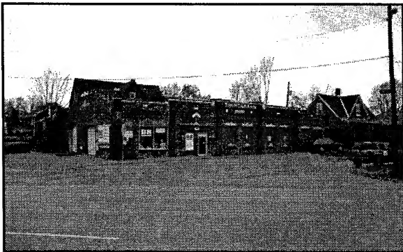
Commercial buildings at 4030 South 13th Street (DO09:0103-003)
